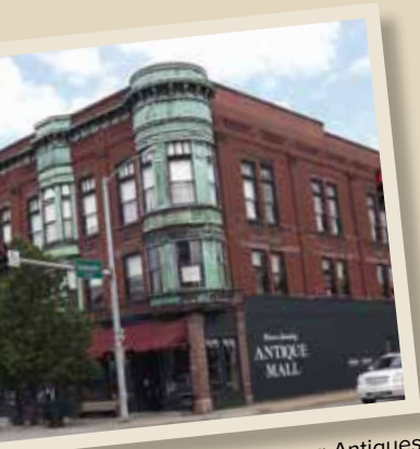
The Galesburg Antiques Mall Company, Galesburg
